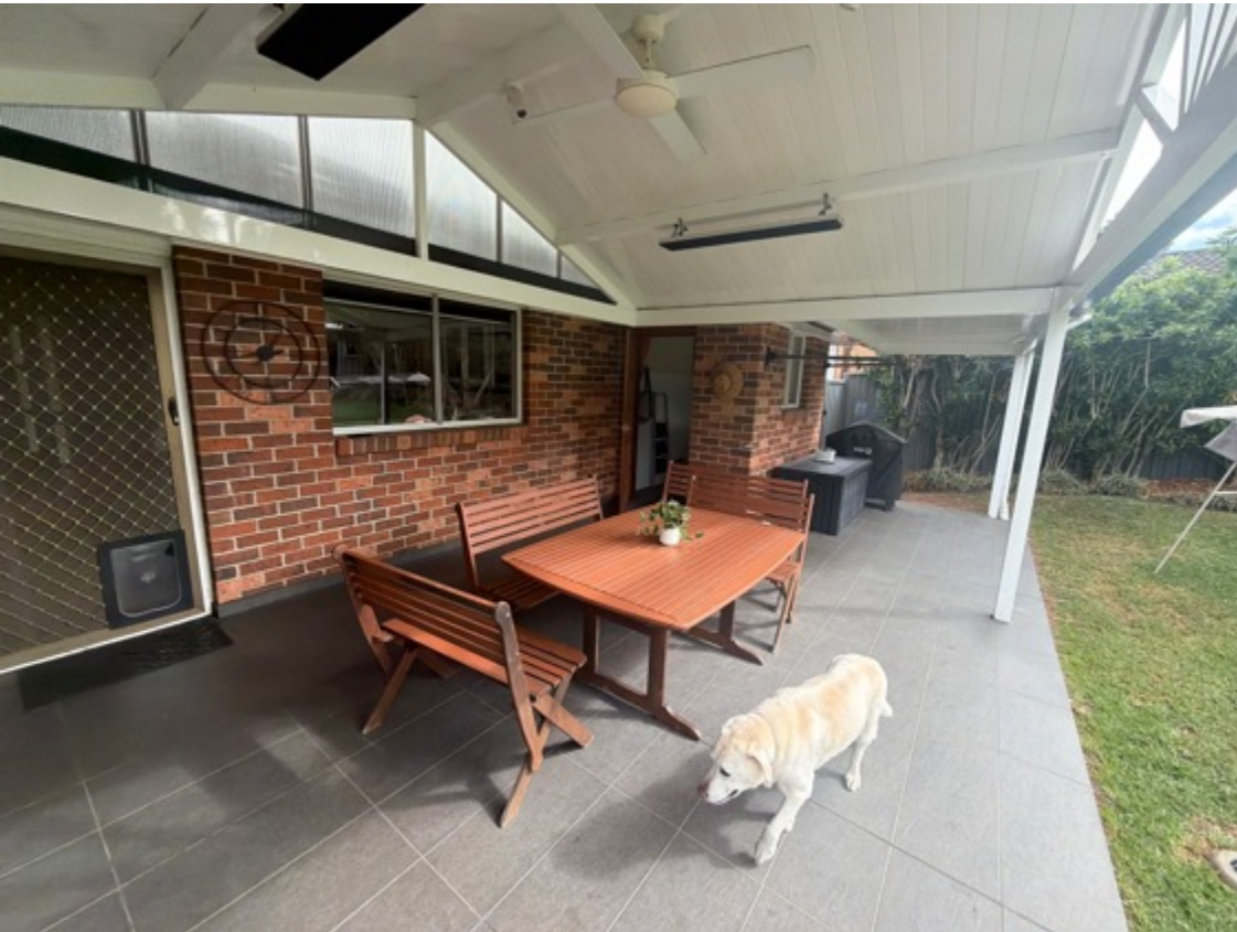
The rear pergola checked is structurally sound.
