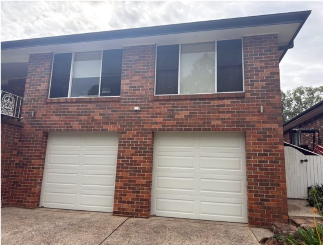
Garage roller doors tested, functioned at the time of inspection.
