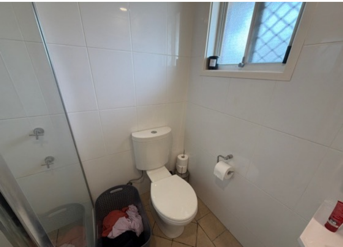
The toilet tested, functioned at the time of inspection.
