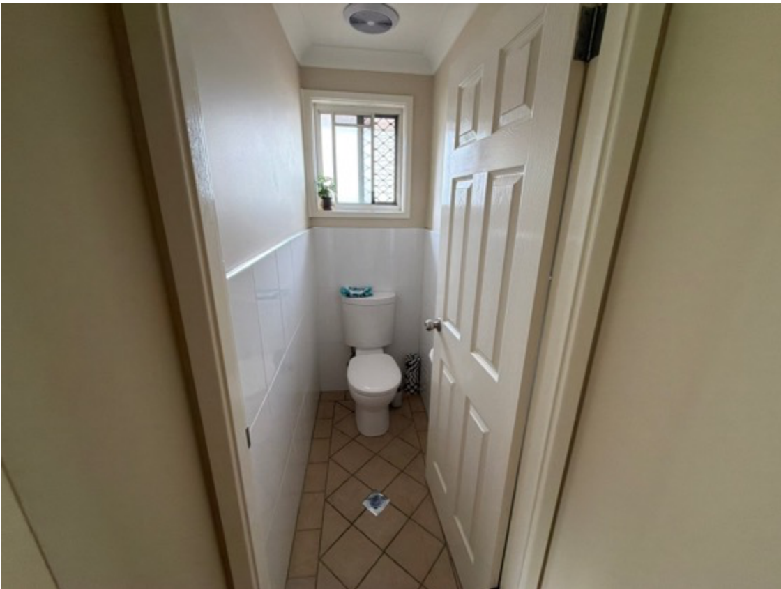
Common toilet water services tested, functioned at the time of inspection.
