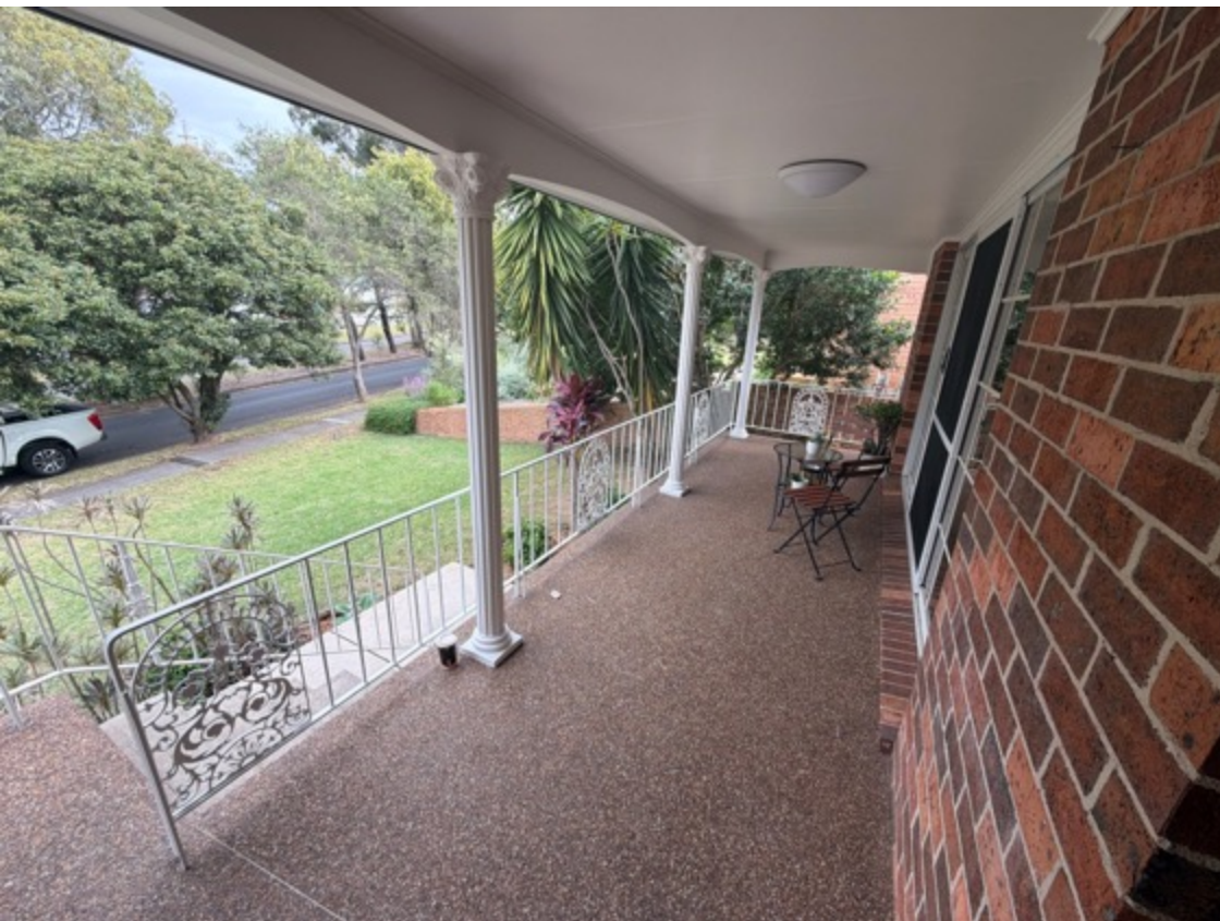
Exterior railings checked are structurally sound.
